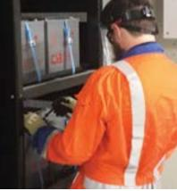
Selecting the battery system deployed with a UPS solution is a significant consideration. With larger UPS systems, the battery can contribute up to 50% of the cost and 100% of the back up power. This article explores the key considerations in
